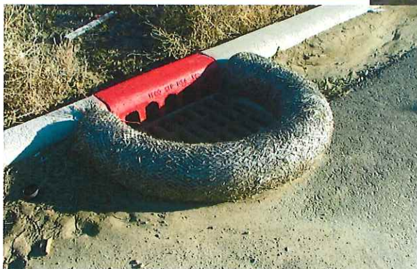
Straw wattle installed at stormwater inlet.
