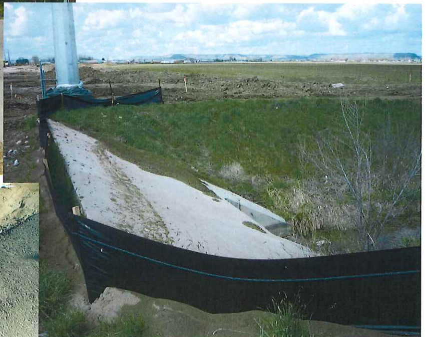
Properly installed silt fencing.
