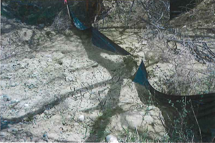
Improperly installed and unmaintained silt fencing.
