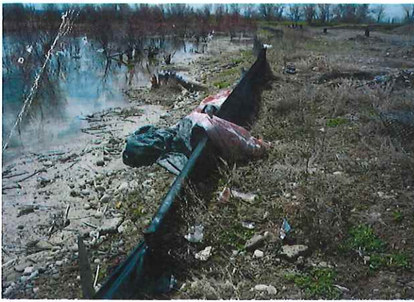
Improperly installed and unmaintained silt fencing.
