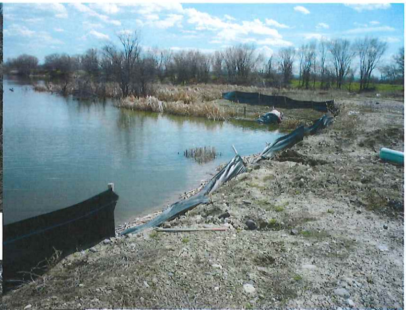
Improperly installed and unmaintained silt fencing.
